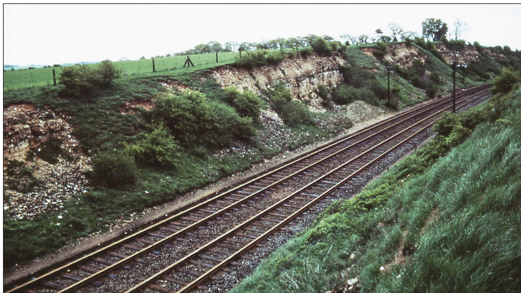
Figure 11. Ancaster railway cutting, showing cambered Lincolnshire Limestone; the slumped, vegetated sections mark parallel 'gulls' (fissures opened by 'stretching' of the limestone and filled with soliflucted and colluvial materials) transected by the cutting (view E at SK 995443, April 1968)
